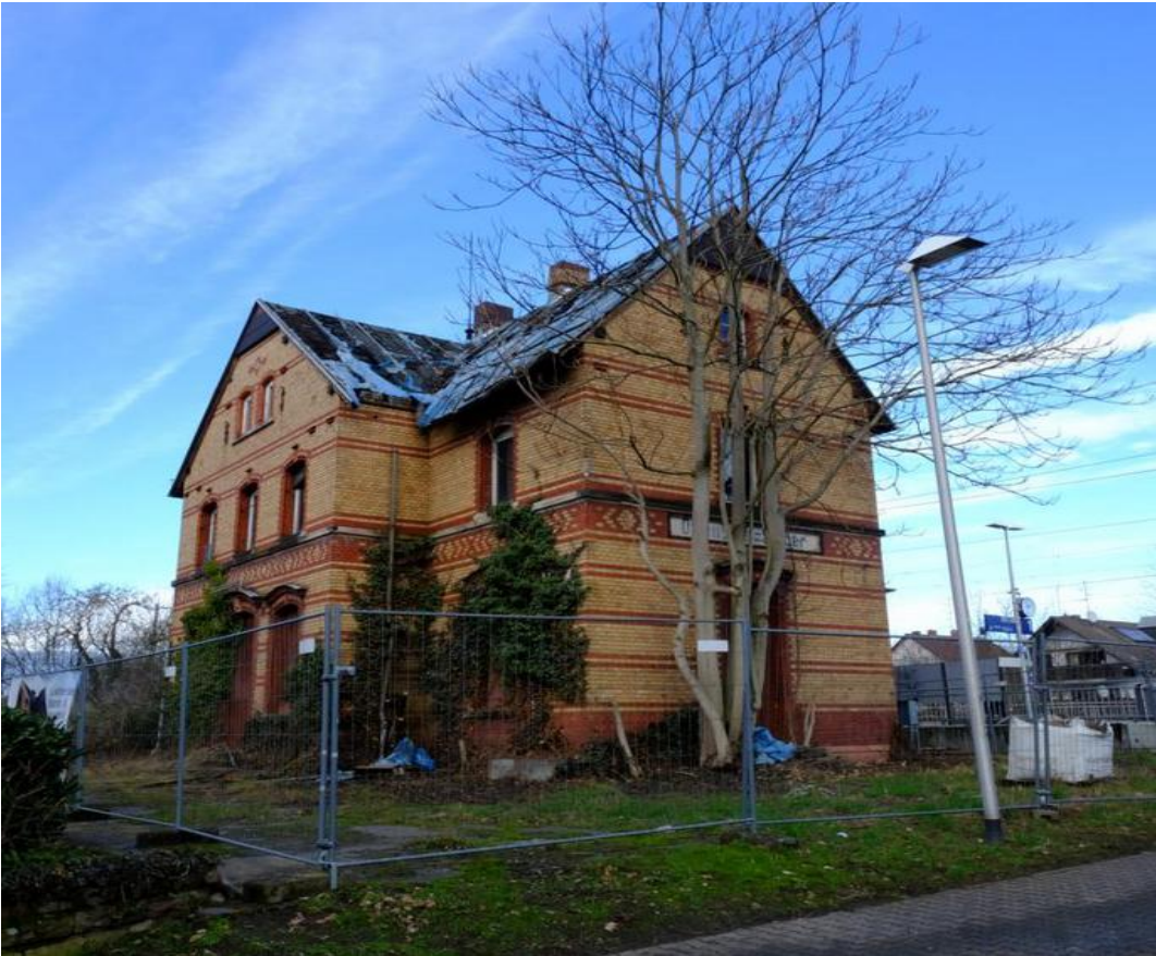
Station Offenbach-Bieber, S1+2
